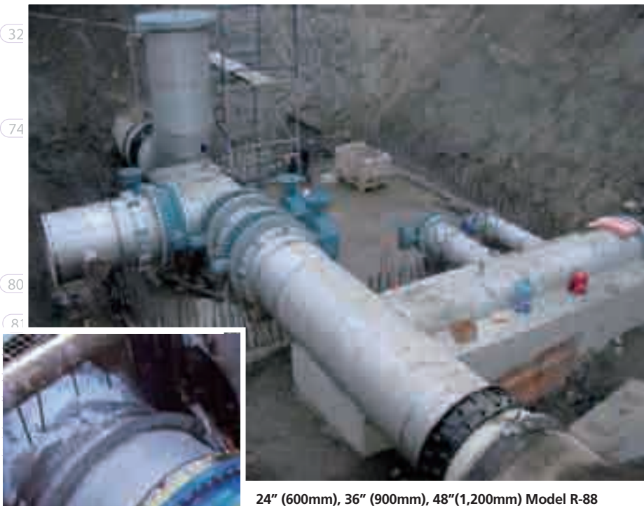
24" (600mm), 36" (900mm), 48" (1,200mm) Model R-88 couplings with stainless steel rings used on stainless steel hydro electric pipe line, Vernon, British Columbia, Canada
