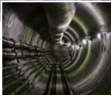
12" (300mm) & 14" (350mm) R-88 couplings used in tunnel boring / mining application. The pipe line delivered a bentonite water mixture while the outflow was an aggressive rock and mud slurry, Portland, Oregon, USA
